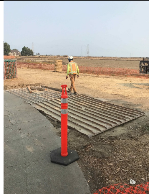
Construction entrance installation at Sea Cloud Park Staging Area
