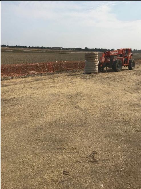
SWPPP measure installation at Sea Cloud Park Staging Area
