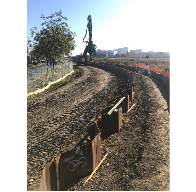
Sheet piles being adjusted to final grade near ~Sta. 340+00
