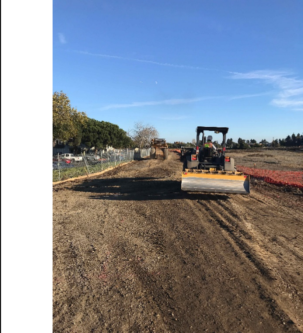
Equipment grading/clearing the trail near ~Sta. 340+00
