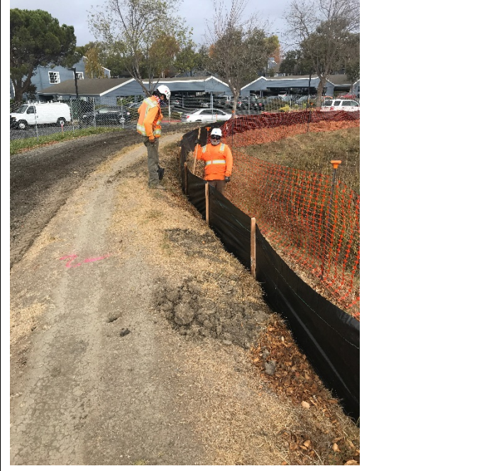
Installation of silt fence & ESA fencing near ~Sta. 340+00
