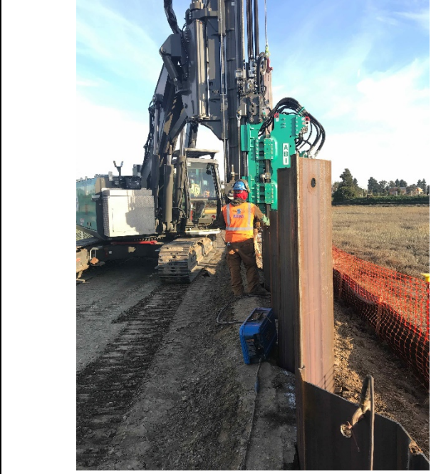
Sheet piles being installed
