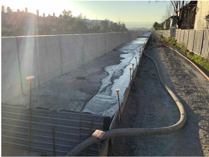
Lightweight cellular concrete fill placement at FW 19 in Phase I
