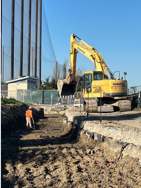
FW 3 subgrade excavation near Mariner's Point Golf Center in Phase III
