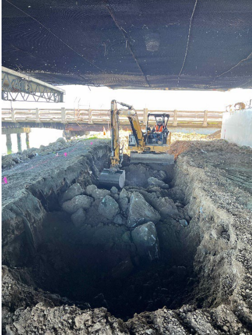
Excavation for FW 25 below the San Mateo Bridge
