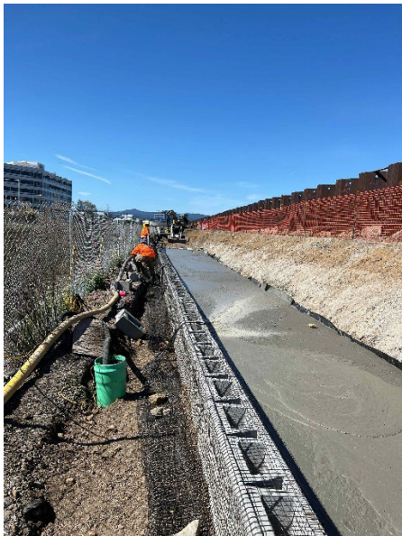
Lightweight Cellular Concrete and block placement at Retaining Wall 2 near Sta. 93+00
