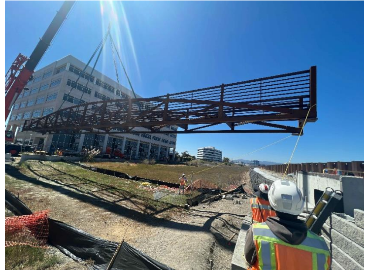
Bridge installation for AP-9 pedestrian bridge near Sta. 85+00 in Phase III
