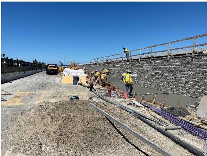
Concrete placement for Access Points in Phase II along Beach Park Blvd
