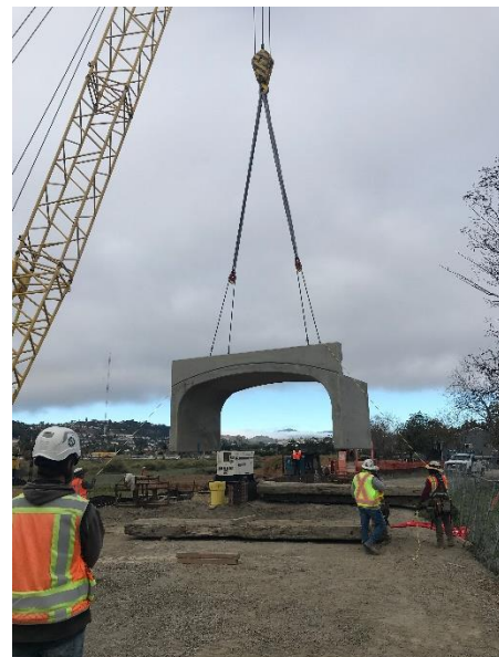
Access Point 42 (Egress Bridge) segment placement near Sta. 331+00 in Phase III
